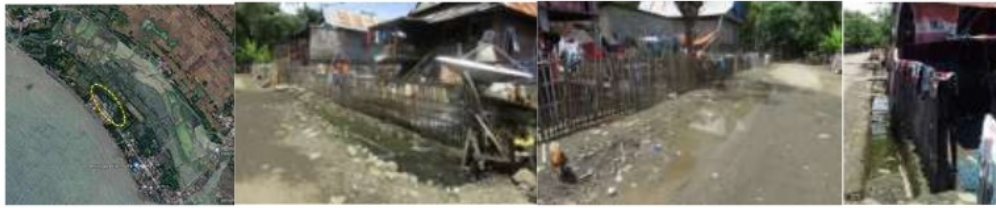
Picture. 5. The drainage system on environmental roads
